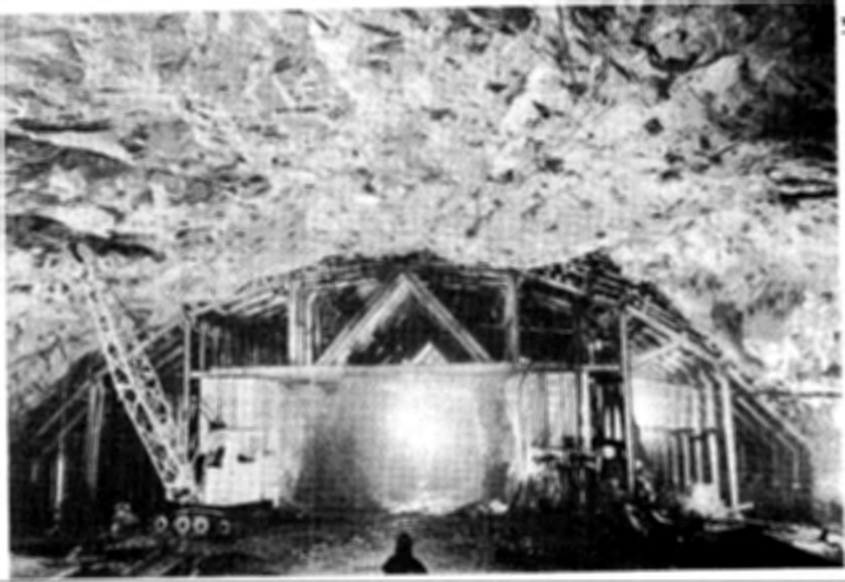
(a) Rock bolting and light steel support September 1956
